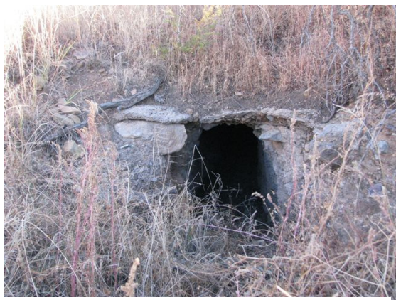
Figure 8. Entrance to 300 foot Tunnel on Dead horse Mesa.
