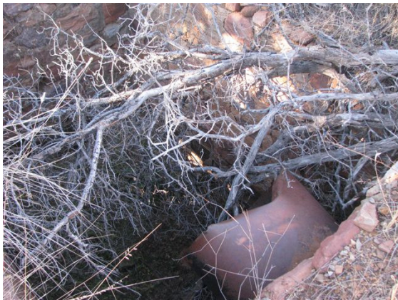
Figure 9. Penstock on Dead Horse Mesa with 20-inch Pipe
