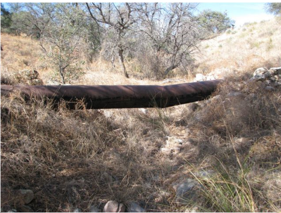
Figure 7. Water Pipeline crossing Arroyo above Apache Springs.
