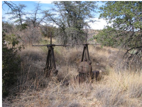
Figure 10. Terminal Valves on Ridge above Boston Gulch
