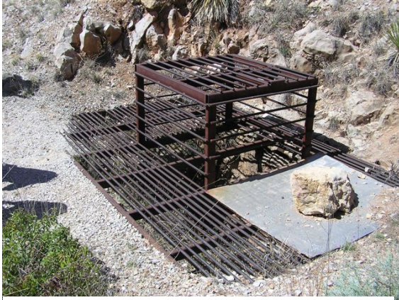
350 Foot Deep Mine Shaft Photo by T. Johnson - 2009
