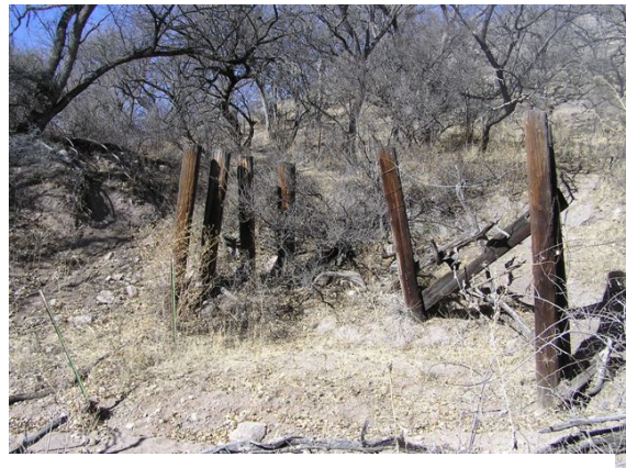
Wood Supports for Railroad Trestle Photo by T. Johnson
