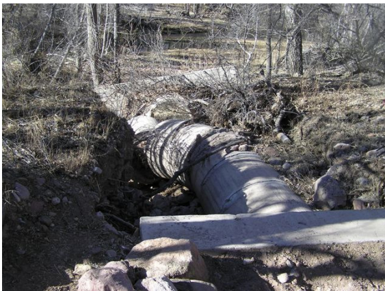
Concrete Culvert through Railroad Bed Photo by T. Johnson
