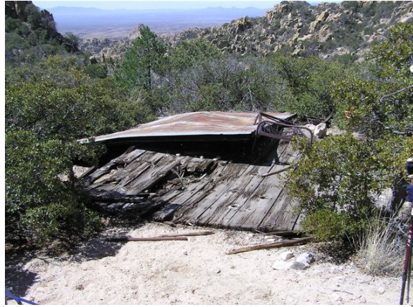
Remains of the control shack that kept track of the ore shipments
