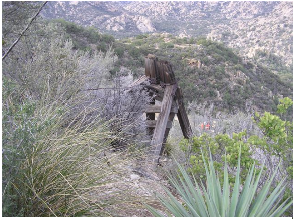
Remains of a pylon used to support the cable car system
