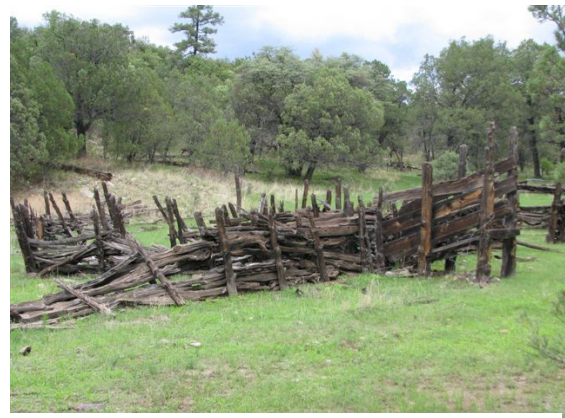
Remains of the Corral and Cattle Loading Ramp
