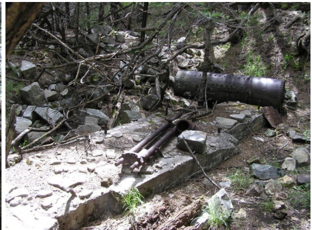
Concrete Base for a Compressor
